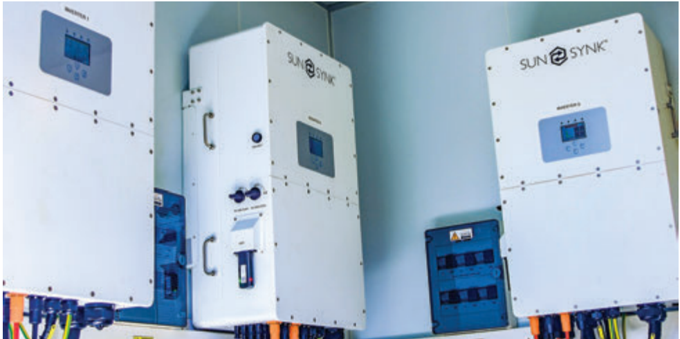
Residentia Sering’s 150kVA PV solar system can provide up to 4-5 hours of backup power, converting sunlight into 240kW of battery energy.
