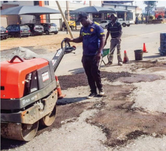
The Tar Paving and Landscaping team working hard to fill the potholes in Waterval Avenue
