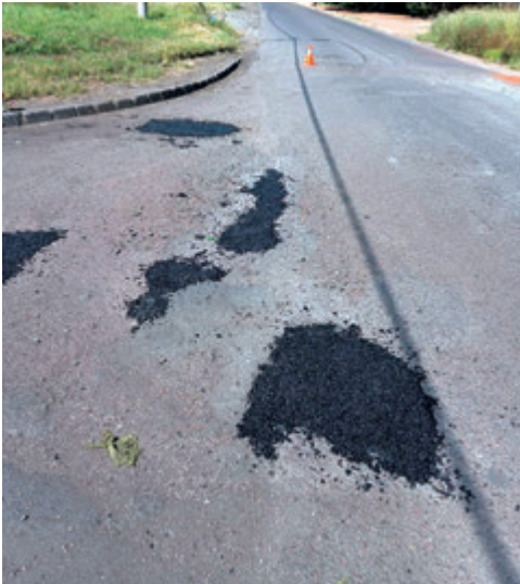
After – CPF sector 5 members filled several potholes in Dawes Street.
