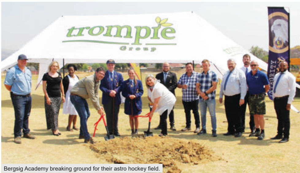
Bergsig Academy breaking ground for their astro hockey field.
