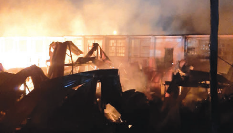
The roof of the warehouse collapsed as a result of the fire.
