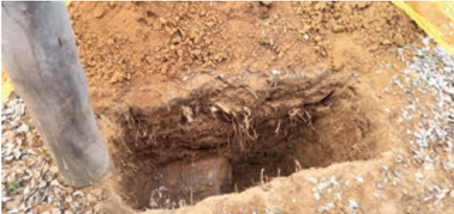
Two men dug the holes with their hands for the poles that needed to be erected.
